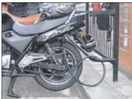
Fig 57: Hitching rail protected by railing to avoid creating a trip hazard to pedestrians. Source: Department for Transport.
